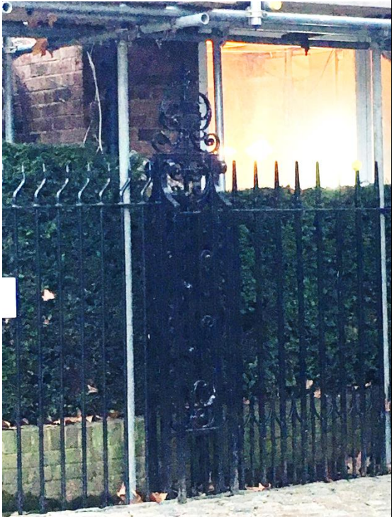
Existing Decorative Piers.
