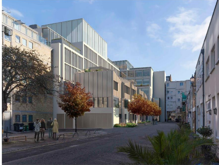
View to rear of building within Chilworth Mews - Consented
