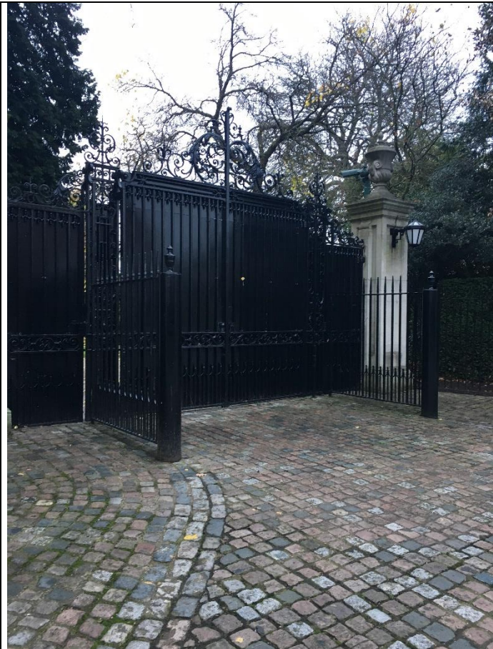
Existing Entrance Gates.
