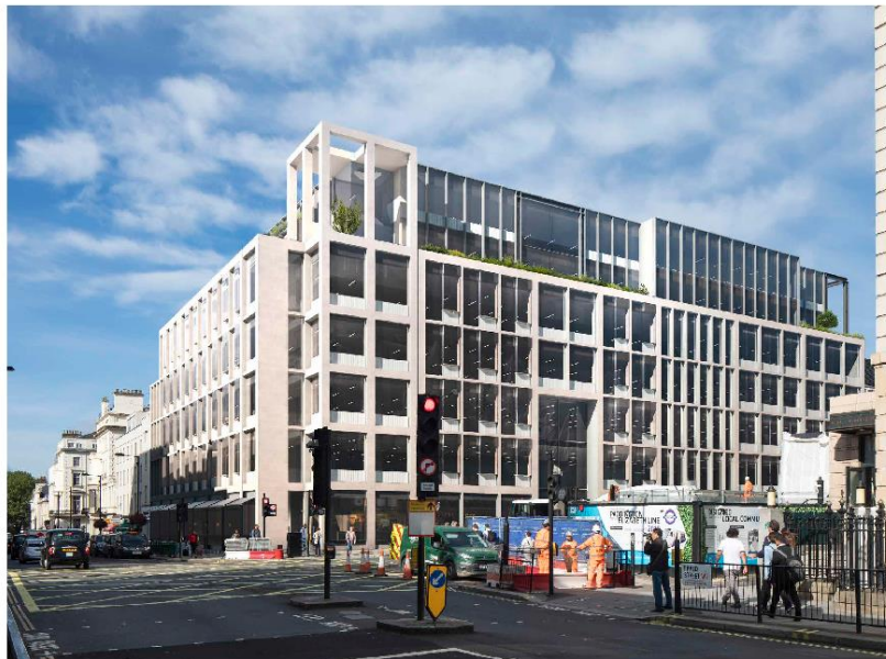
Approved montage from Eastbourne Terrace and Craven Road junction (top) and as proposed (bottom).
