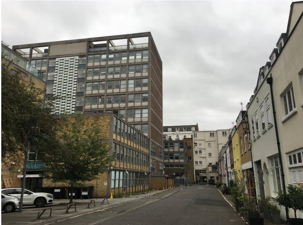
Front elevation at junction of Praed Street, Craven Road and Eastbourne Terrace (top) and rear of site in view along Chilworth Mews (bottom).
